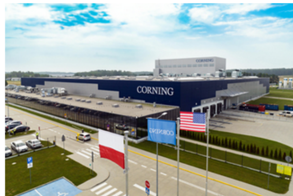
Pole of excellence: Corning's new fiber facility is one of the largest in the EU.
