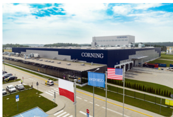
Pole of excellence: Corning's new fiber facility is one of the largest in the EU.
